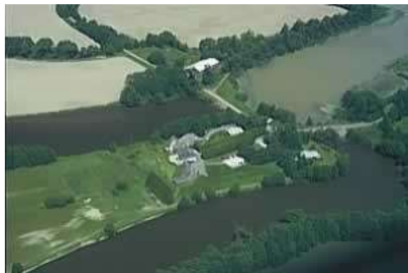
Aerial view of Alaksen NWA buildings 2002.
