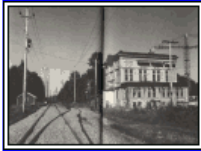
The Coghlan Substation (pages 192 & 193)
